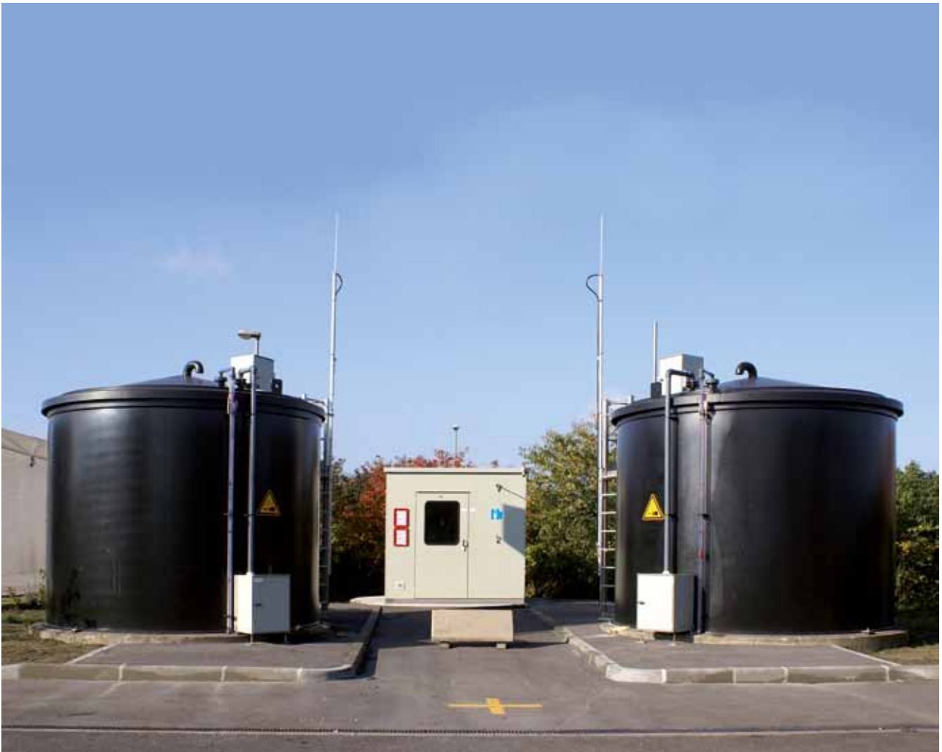
Fig. 3 : Tank and metering station
