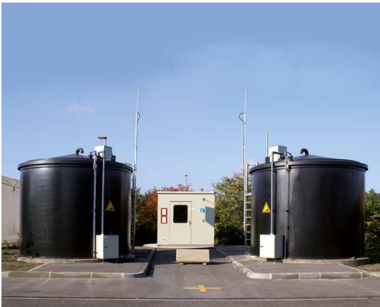
Fig. 3: Reservoir et station dosage
