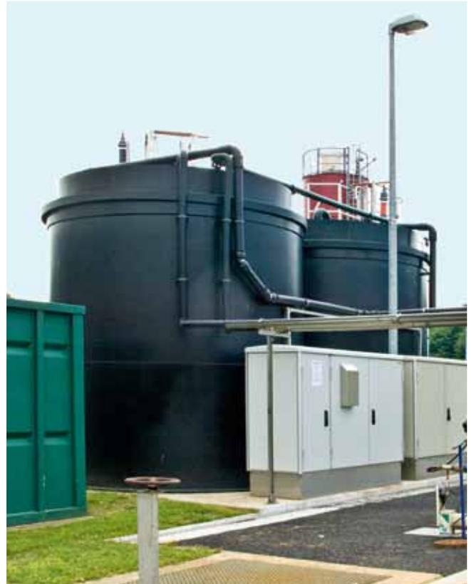
Fig. 5: Storage and metering station for liquid iron salts
