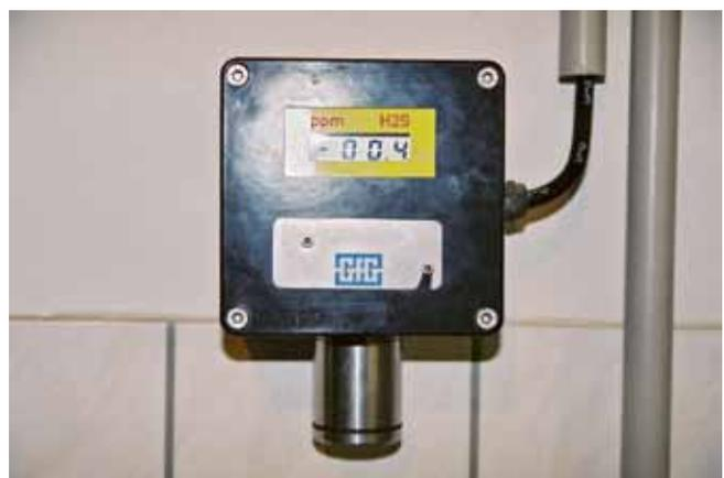
Fig. 8: An H<sub>2</sub>S sensor takes continuous readings in the grit chamber. The signal is processed and the KRONOFLOC metering pumps activated. The results are illustrated in Fig. 10.
