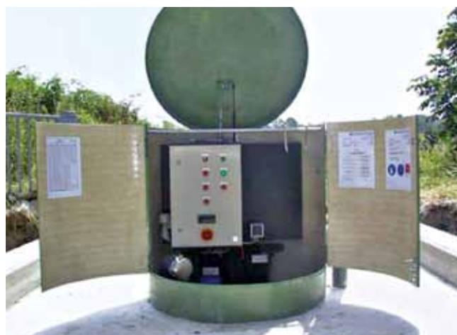
Fig. 3: Metering station in a manhole
