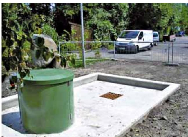
Fig. 2: Underground tank at a pumping station with catch basin
