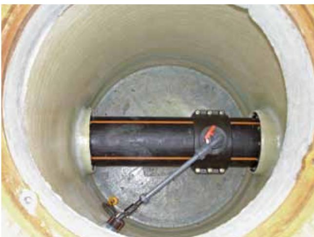
Fig. 5: Addition directly into the pressure pipeline via a seeding point.
