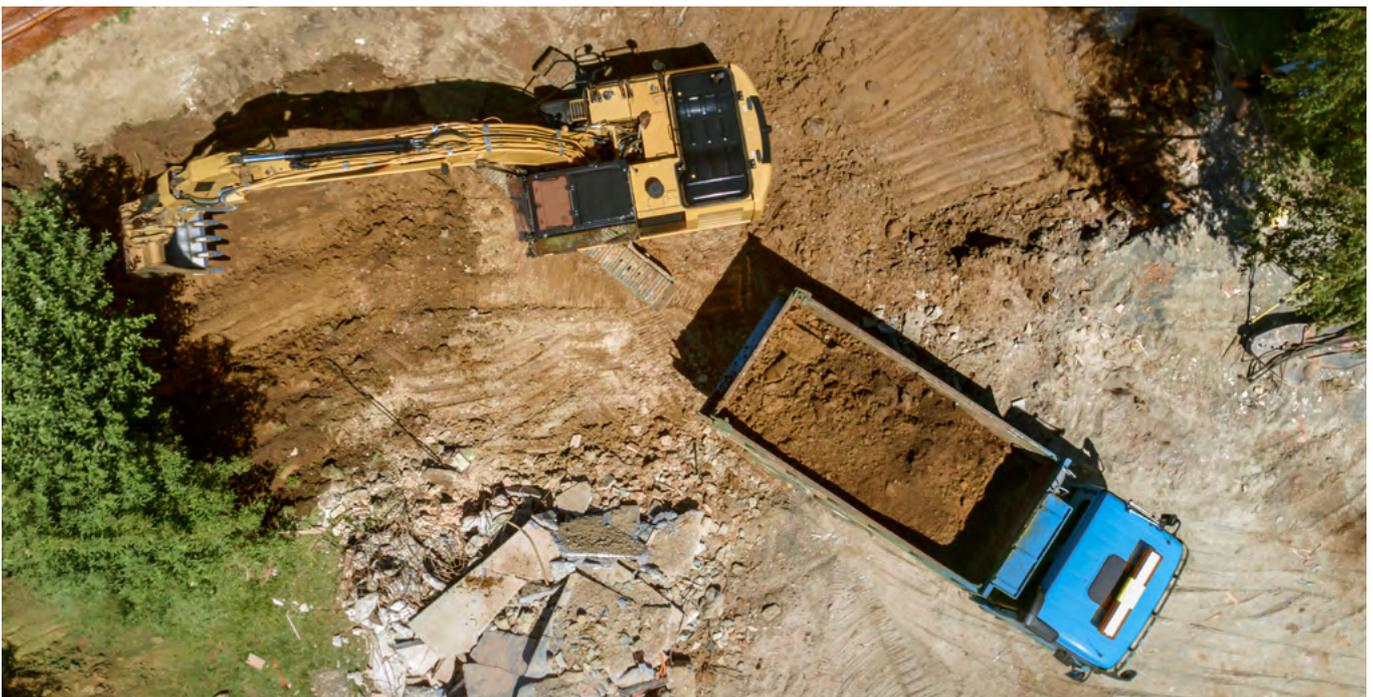
Fig. 3: Soil removal as part of remediating a contaminated site
