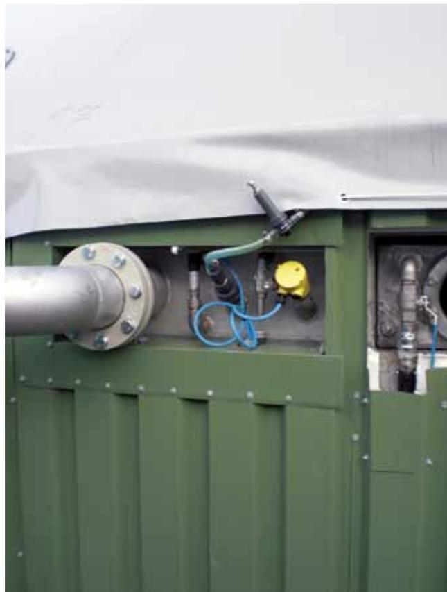
Fig. 2: Possible points of addition for iron salts – mixing tank (left) and straight into the fermenter (right)
