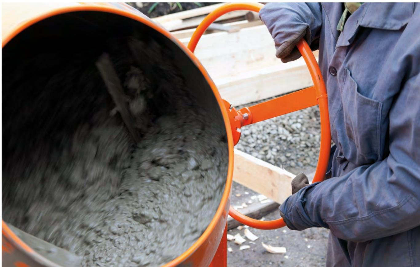
Depending on the origin of the raw materials used and the clinker production conditions, cement contains up to 100 ppm hexavalent chromium (chromate). In this water-soluble form, chromium is capable of penetrating the human skin and can cause an allergic reaction known as chromate dermatitis, depending on the intensity and duration of exposure.
